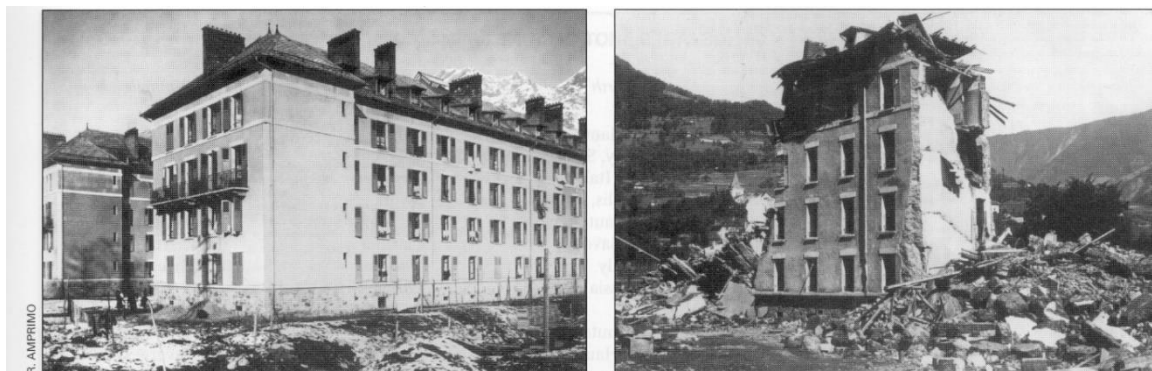
Left: The three apartment blocks at Les Corrues had been built on a design drawn up by Charles Fourier, a French 'utopian' philosopher of the 19th Century. Fourier advocated that care and co-operation were the secrets of social success and he devised apartment complexes where people should ideally live, the so-called 'Phalanstères'. Fourier's ideas led to various
